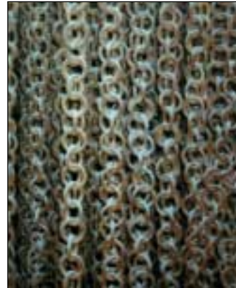
Chain System After Retrofit
